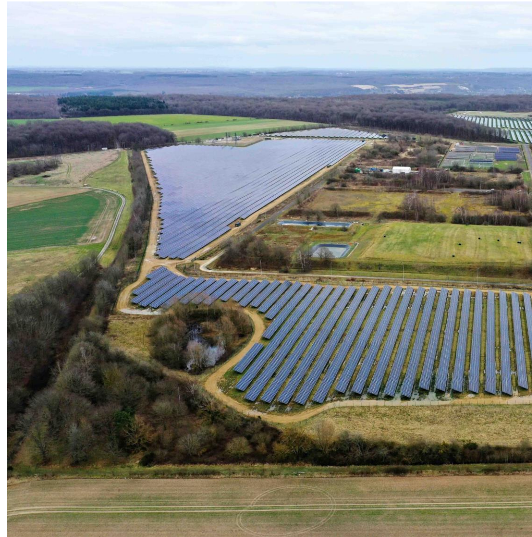
Solar panels, France (CVE Group).
