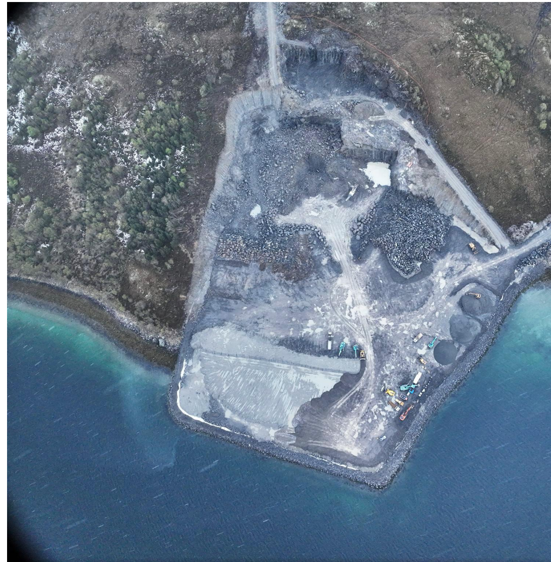
Biogas unit in Norway, ready for construction to begin (FDE).
